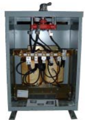
Secondary Loadbreak Switch for multiple Heater Voltages/Stages
